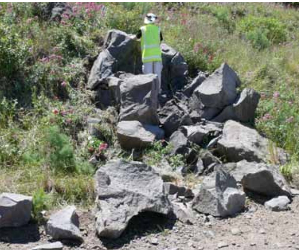
A large rock reduced to a jigsaw of pieces by Nonex.
