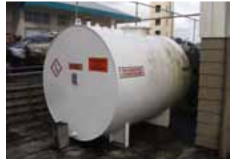
Diesel tank showing NON-HAZARDOUS CONTAIN SPILLAGE on side and a ECOTOXIC diamond on the front, at least the correct diamond is showing.
