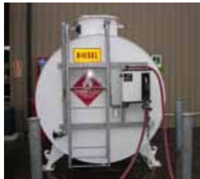
Diesel tank showing NON-HAZARDOUS CONTAIN SPILLAGE on side and a Flammable Class 3 diamond on the front.
