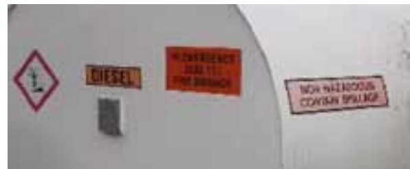
Diesel tank showing NON-HAZARDOUS CONTAIN SPILLAGE on side and a ECOTOXIC diamond on the front, at least the correct diamond is showing.
