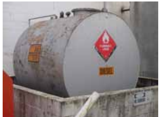
Diesel tank with a red Class 3 diamond and UN 1270. UN 1270 is for an obsolete number for PETROLEUM FUEL.
