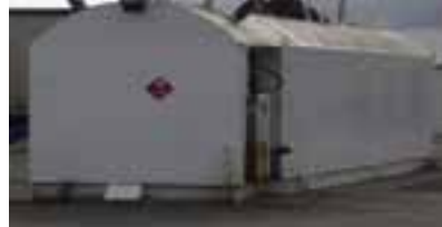
Diesel refueling tank with a red 3.1D Flammable Liquid diamond!
